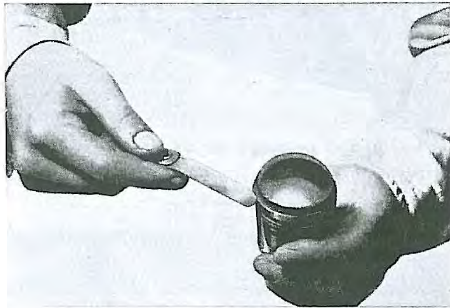
Fig. 56. Measuring clearance between piston ring groove and ring
